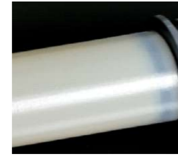
管材焊接 Pipe welding
